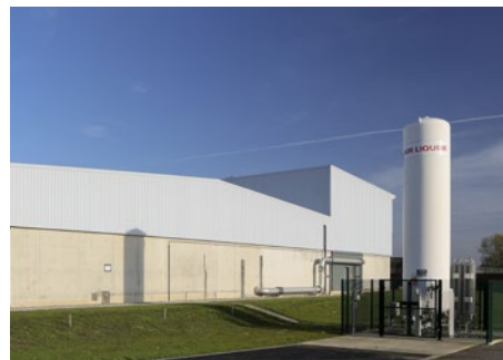
View of Acomb Landing plant with the LOX-tank that feeds the ozone generators.
